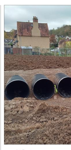
port manifold. The inlet pipe connects into the upstream end of the first pipe only, which effectively converts the first pipe into the primary, combined carrier and storage pipe, with the remaining six pipes functioning as secondary storage pipes at times of peak discharge.
